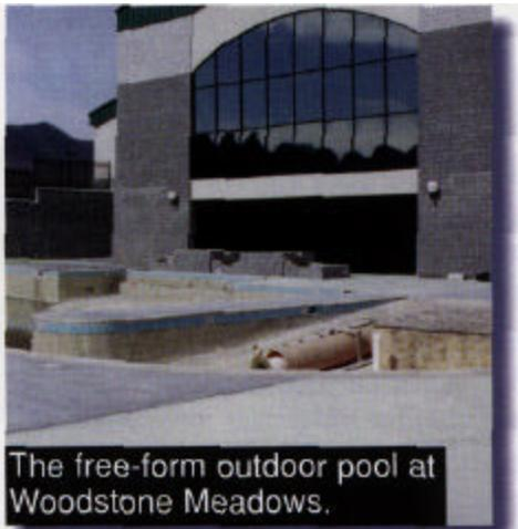
shaped pool consists of a shallow, 18inch entry on one leg of the Z, a 25meter pool in the middle portion and a 10-foot-deep diving well on the other leg. The 8- to 18-inch-deep wading pool also features a children's play fountain.
